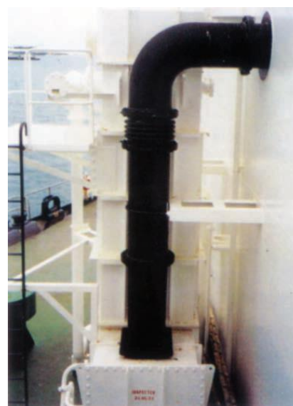
Inert gas line coated with T-GUARD
